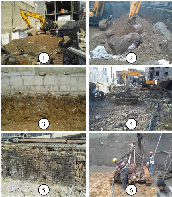
Figure 3. The execution steps of the excavation
